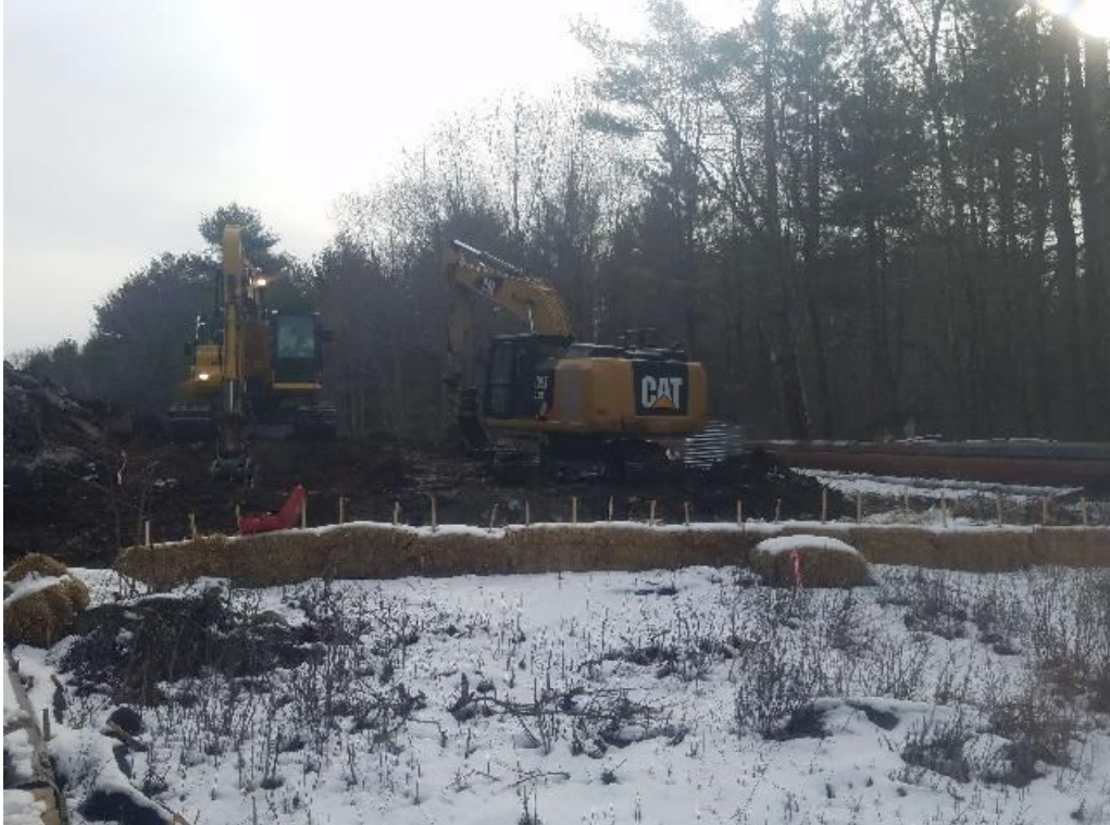
Fig 15: Crew continues to hammer ledge at Str. 75. Viewing east. (03-25-20).
