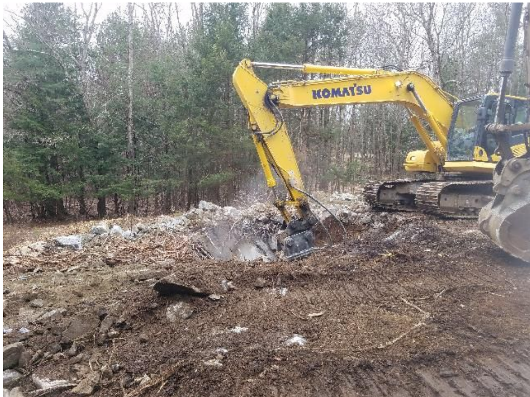
Fig 8: Crew hammering ledge at Str. 74. Viewing south. (03-23-20).
