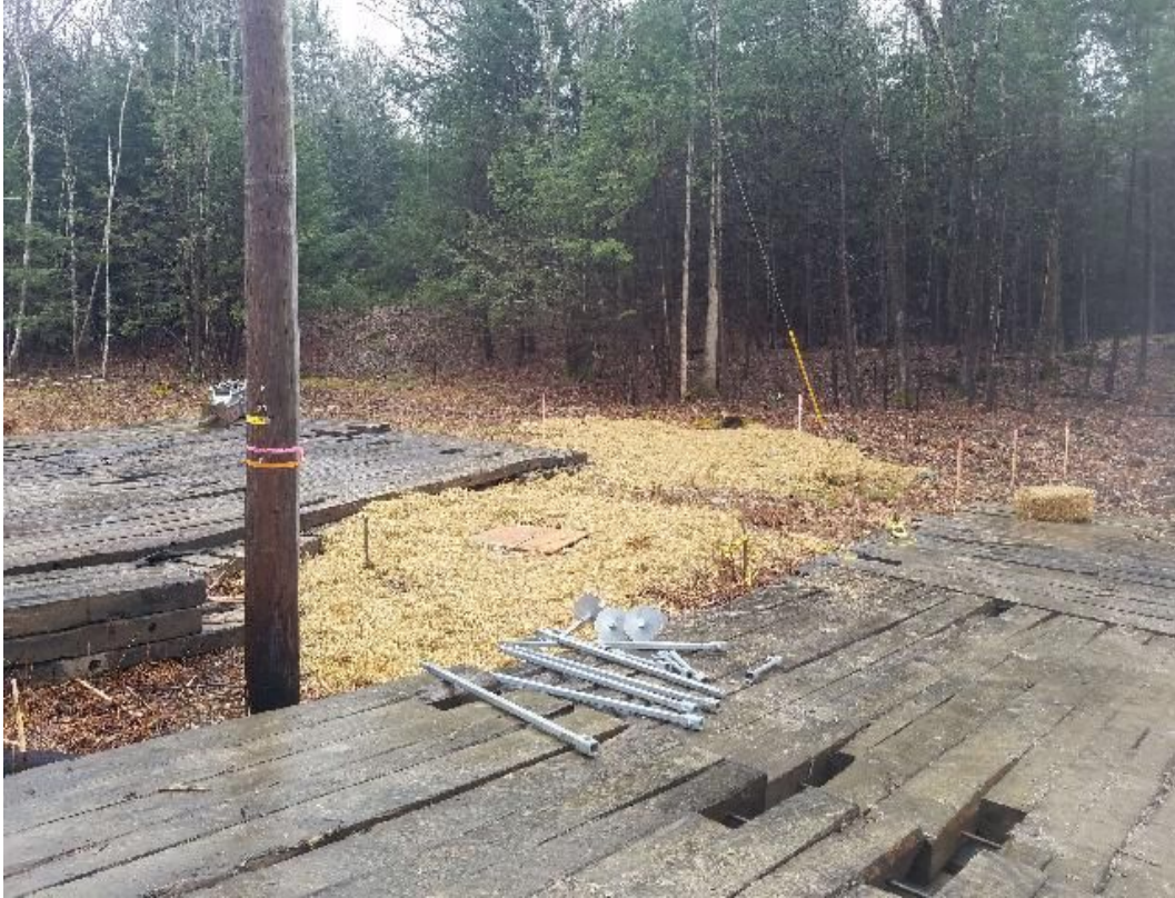
Fig 5: Foundation cans set at Str. 97. Viewing south. (03-20-20).
