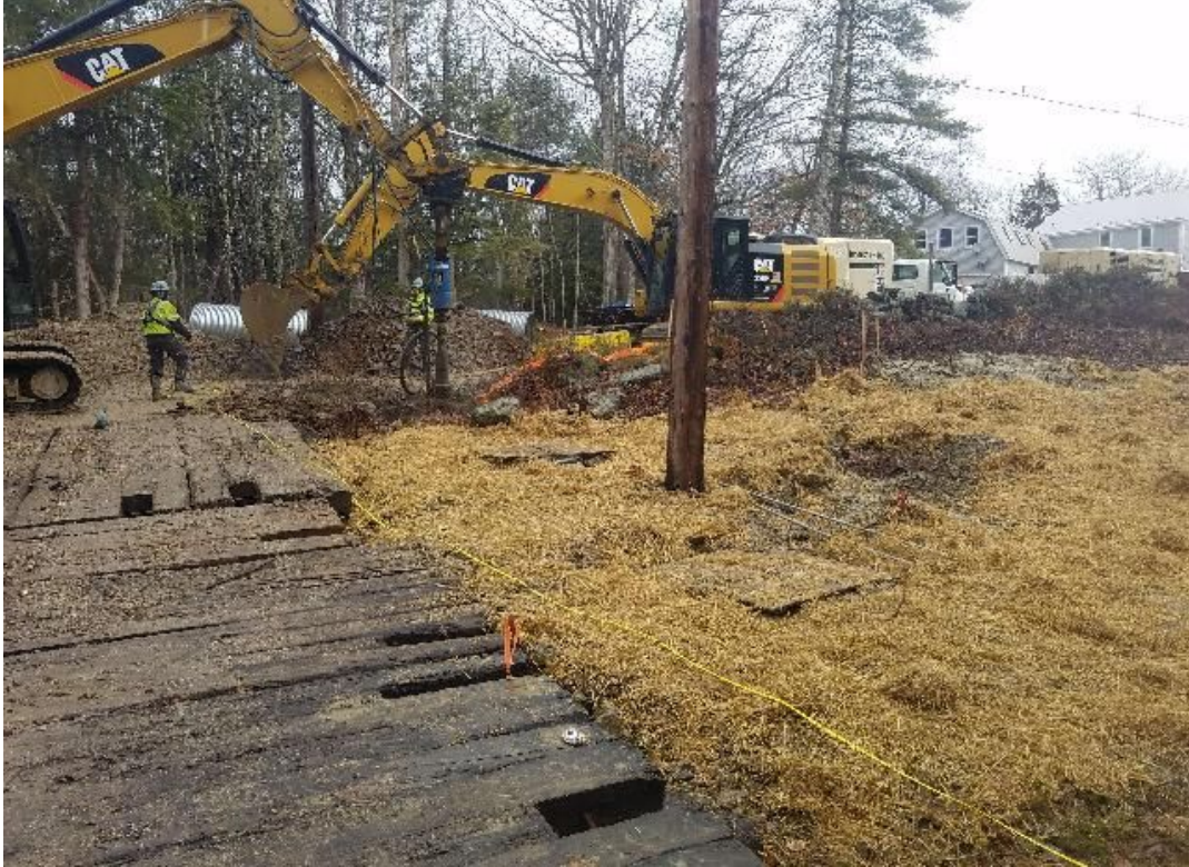
Fig 3: Foundation cans set at Str. 98. Viewing north. (03-19-20).
