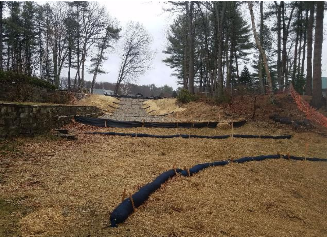
Fig 2: BMPs on slope at Gundalow landing/east side of the Bay. Viewing east. (03-19-20).
