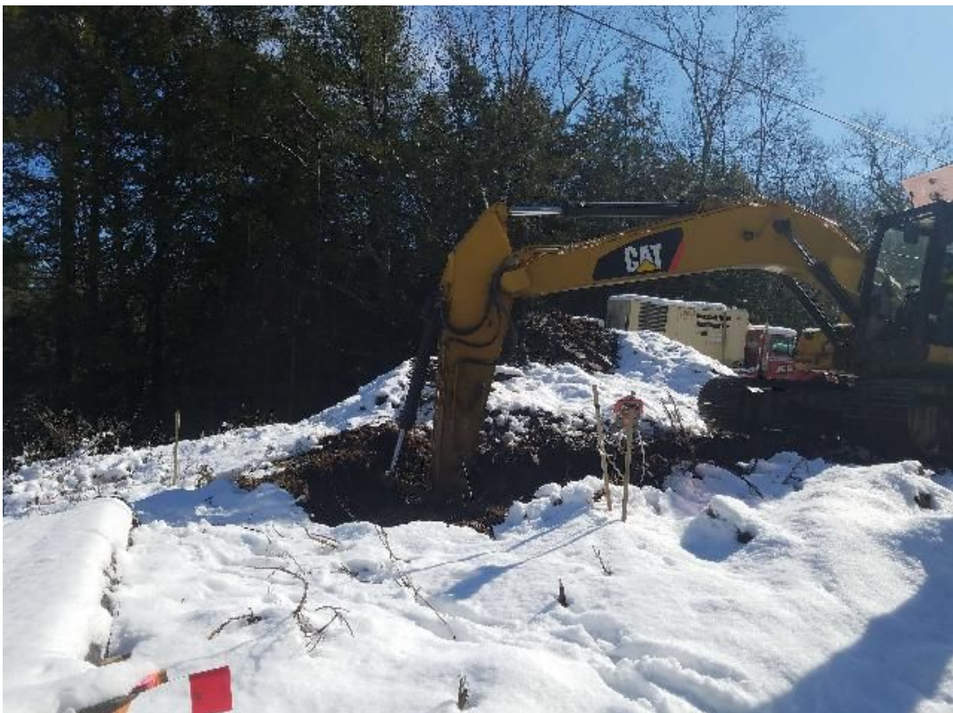
Fig 10: Hammering ledge at Str. 96. Viewing north. (03-24-20).
