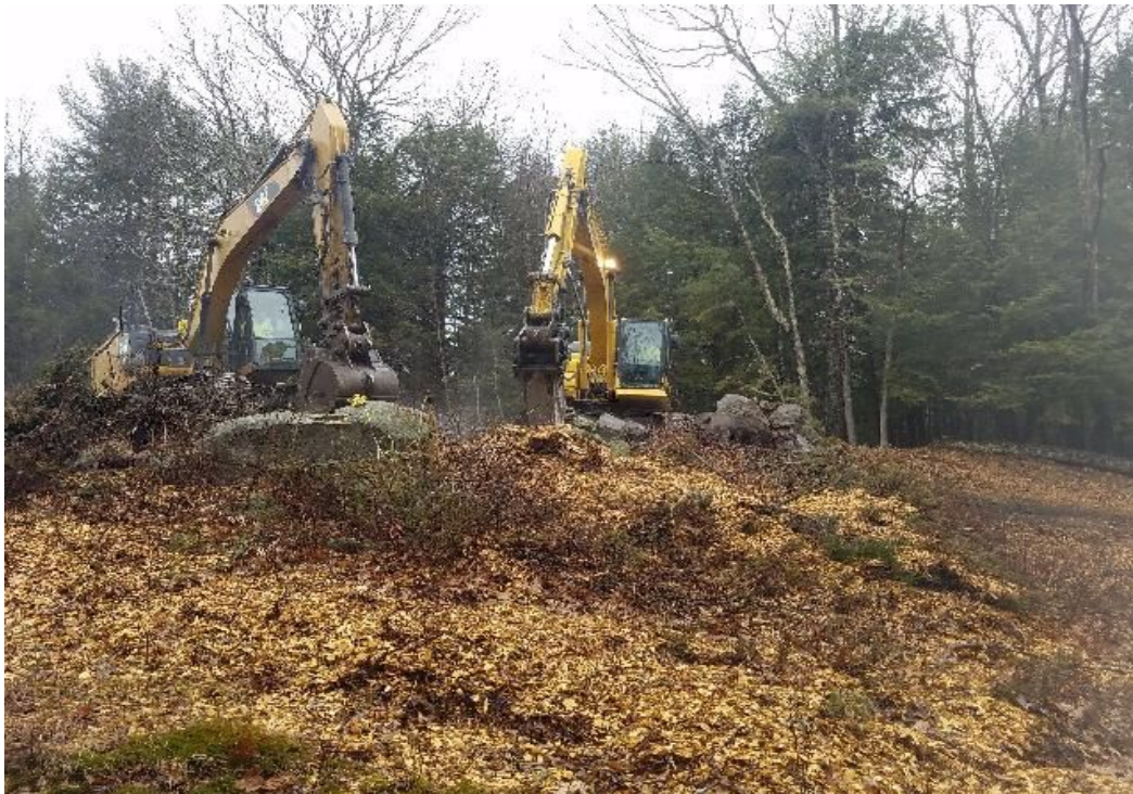
Fig 4: Crew beginning to excavate foundation for Str. 74. Viewing east. (03-19-20).
