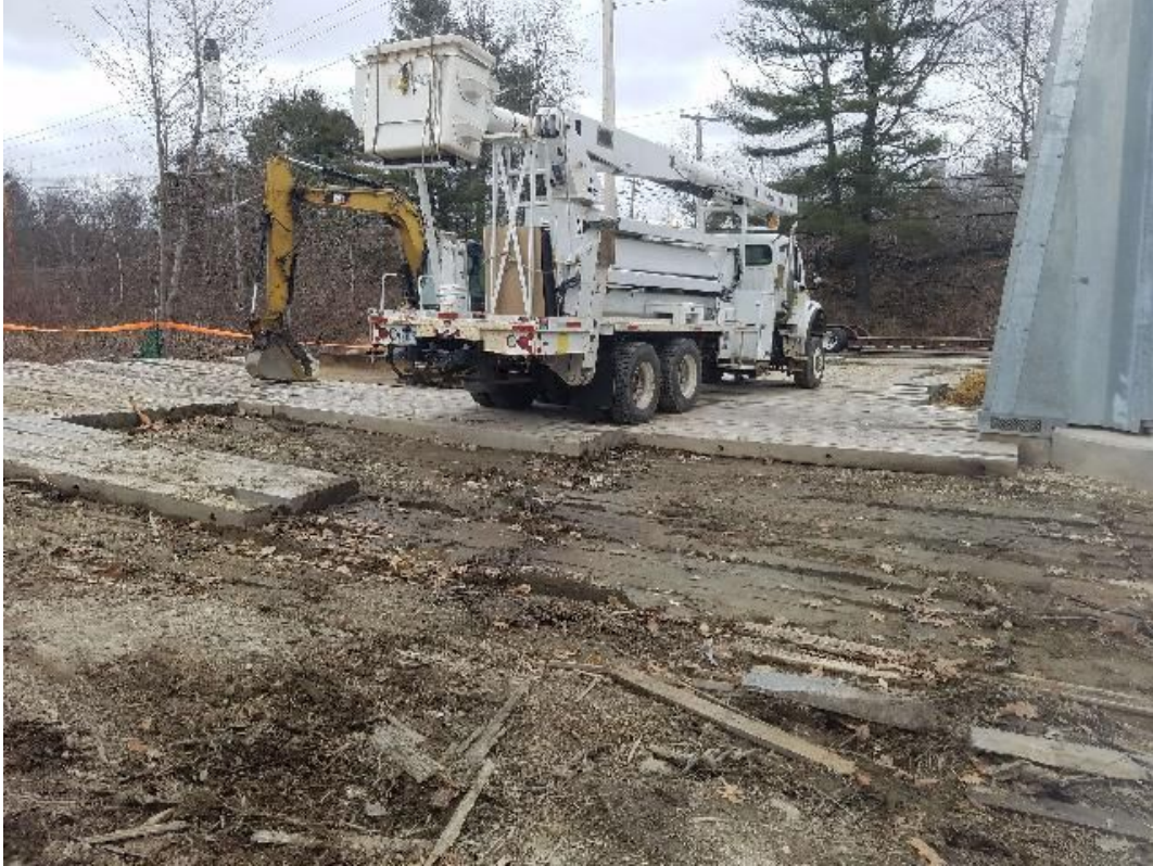
Fig 9: Beginning to remove timber mats at Str 23. Viewing east. (03-23-20).
