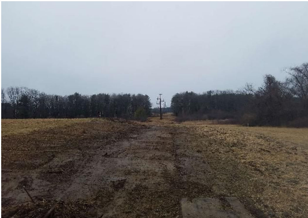
Fig 6: Removing timber mats at Frink farm. Viewing west. (03-20-20).
